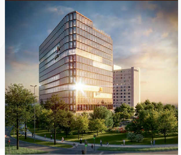
Eclipse building – Germany
